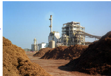
21 MW Tracy Biomass Plant
